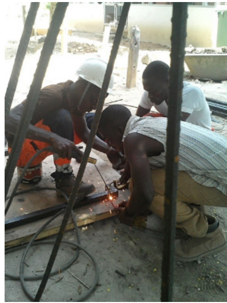
Figure 10 (G): Tacking and welding of iron rod
