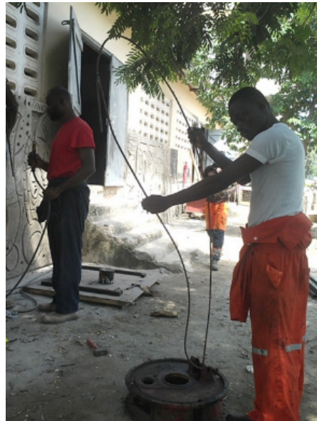
Figure 10 (E): Testing of bent iron rod
