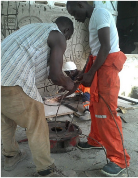
Figure 10 (F) Curling and perforating of metal base for iron rod
