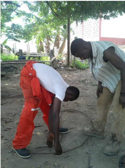
Figure 10 (D): Bending of iron rod on work base
