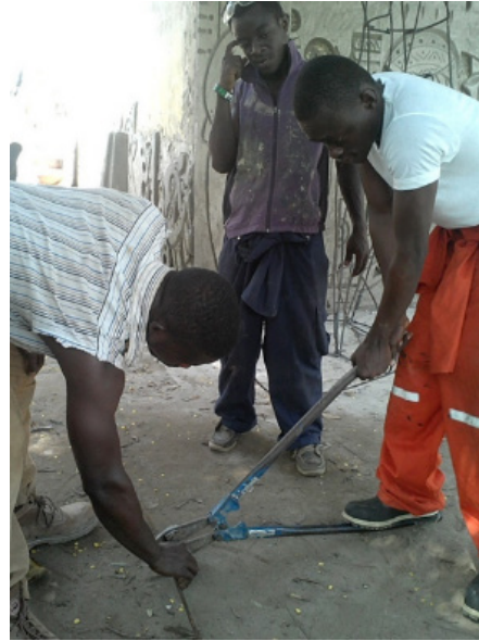
Figure 10 (C): Cutting of iron rods
